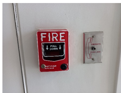
Fire alarm manual station, Fireman phone jack
